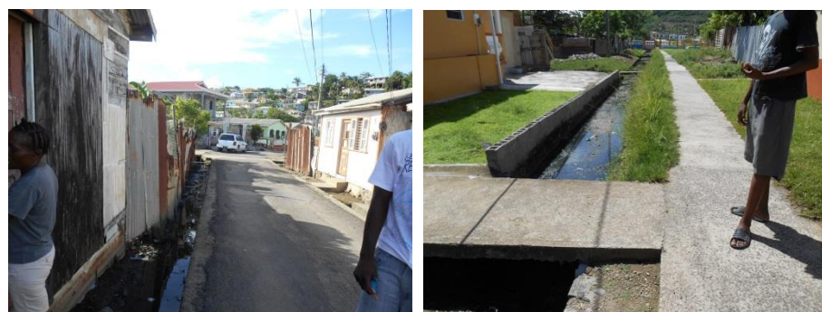
Figure 6-6: Drains filled with silt
