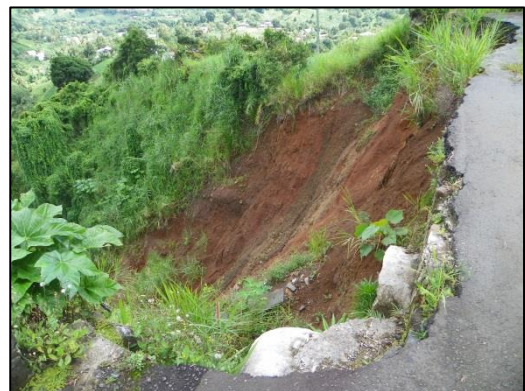
Figure 18. Rockfall and embankment failure in Dominica - Champagne beach area (Left), and Embankment failure in Saint Vincent – Belmont Landslide (Right).
