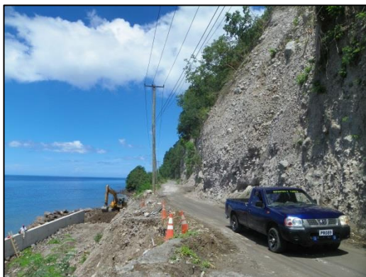
Figure 18. Rockfall and embankment failure in Dominica - Champagne beach area (Left), and Embankment failure in Saint Vincent – Belmont Landslide (Right).
