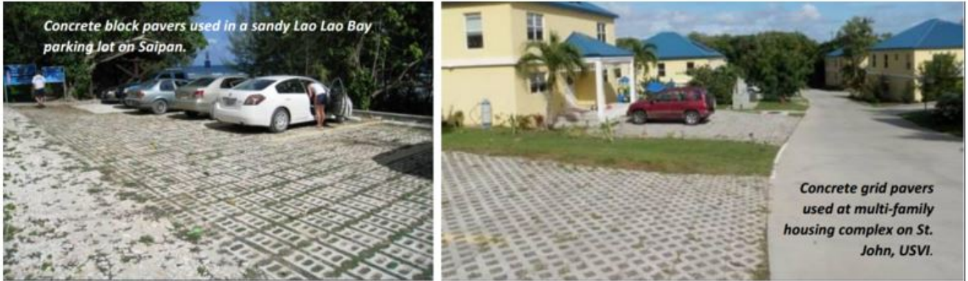
Figure 4: Examples of permeable pavements (Source: Horsley Witten Group, Inc. and Center for Watershed Protection, Inc)
