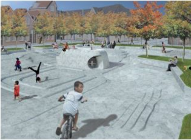
Figure 6: Playground with water storage function (Source: Municipality of Rotterdam)
