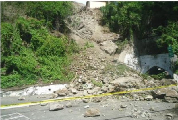
Figure 6: Examples of landslide problems along the road corridors. Upper left: A landslide at the tunnel entrance in St. George, Grenada that happened 21/9/2014. Upper right: A landslide affecting the road from Roseau to the airport, Dominica. Lower Left: Landslide that destroyed primary road in Belmont area, Saint Vincent. Lower Right: Rockfall in road to Stowe, Dominica.
